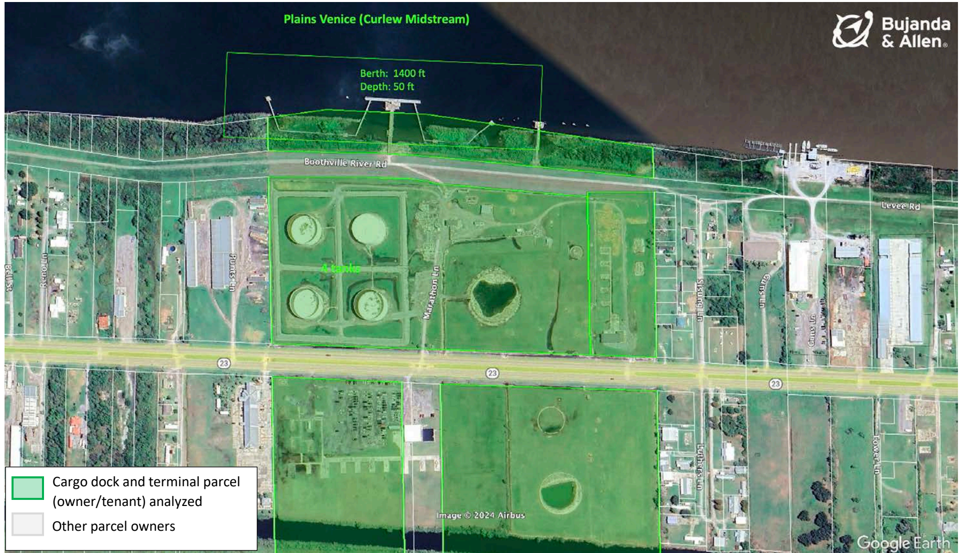
Figure 70. Plains Venice (Curlew Midstream): terminal area and dock.
