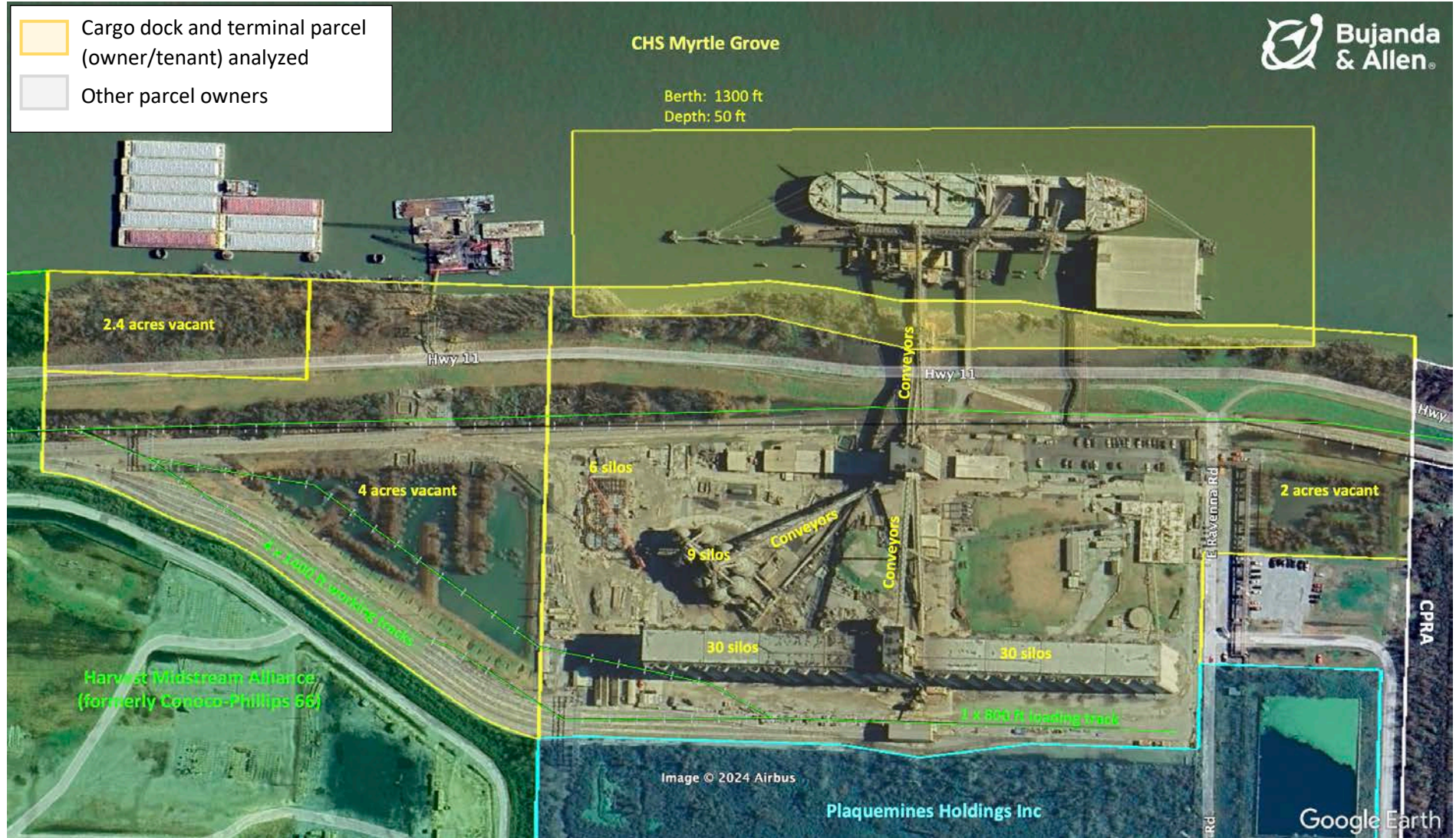
Figure 59. CHS Myrtle Grove: terminal, parcel ownership, dock, and anchorage areas.
